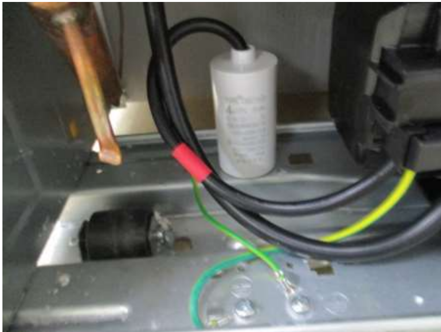
Running capacitor for compressor and earthing terminal
